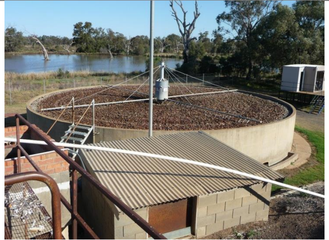
Figure 4.6 – TF No. 2 with amenities building (raised demountable) in background, western side
