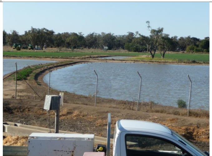
Figure 4.10 – Evaporation Basins (eastern side of plant)
