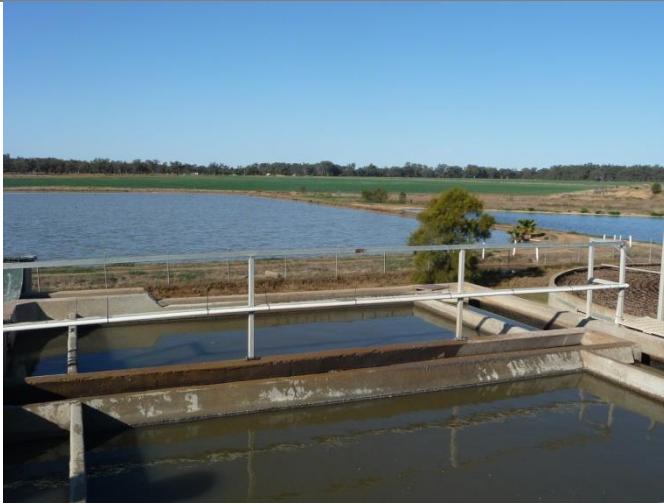
Figure 4.11 – Evaporation Basins (eastern side of STP)
