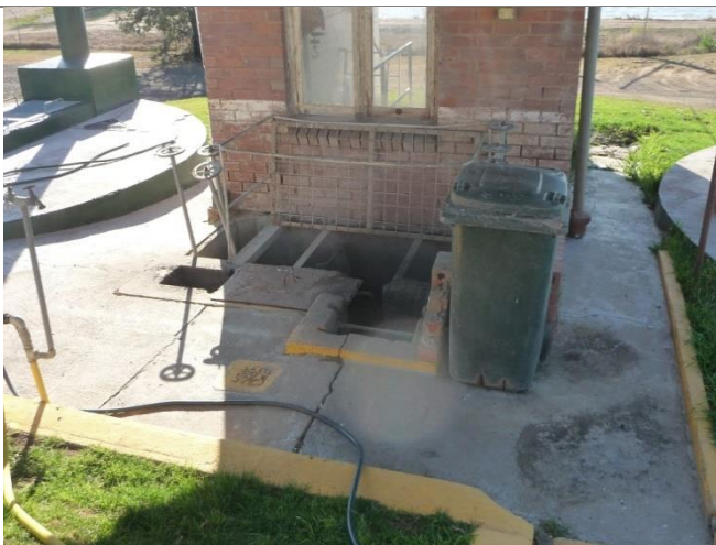
Figure 4.9 – Digester Pump/Mixing Well
