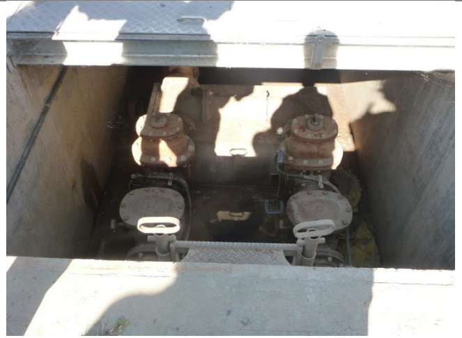
Photo 4.6 – SPS2 Valve Pit
