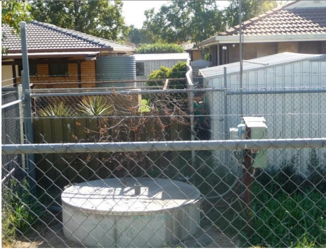
Photo 4.11– SPS4 Wet Well and Switchboard
