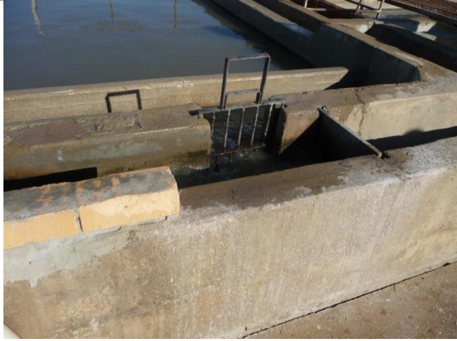
Figure 4.1 – STP Inlet Pit
