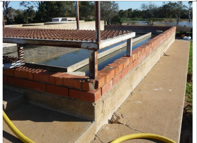
Figure 4.4 – Raised PST wall height
