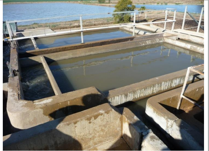
Figure 4.2 – Imhoff Tank
