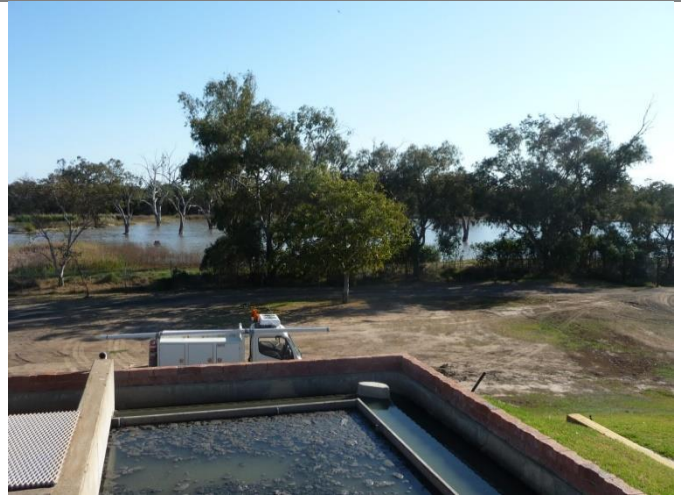
Figure 4.12 – Evaporation Basins (western side of STP)
