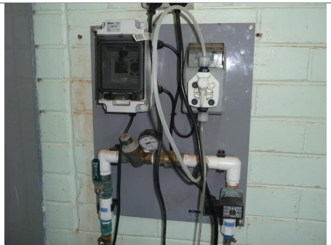
Photo 4.8 – SPS2 Actizyme Dosing Controls
