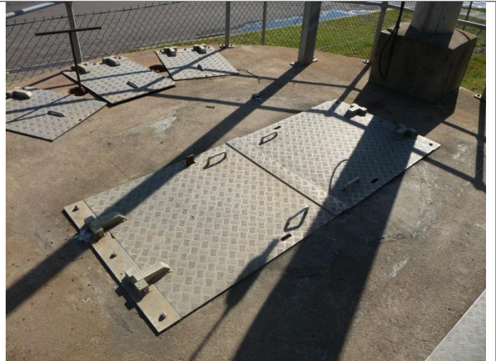
Photo 4.2 – SPS1 Wet Well
